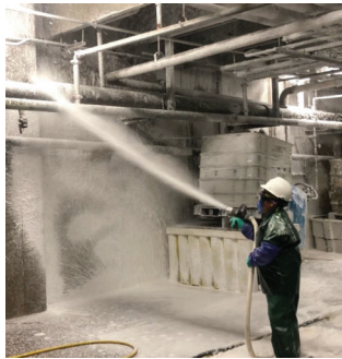
Spectra DF-200 deployed as a stable foam
